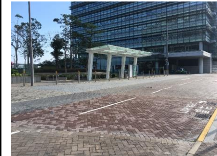
Layby between Building 12E & 16E
