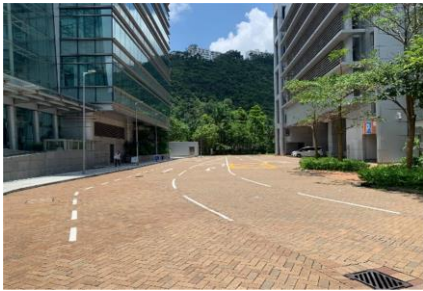
Open Parking Space outside Building 3W
